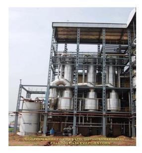
I<sup>st</sup> Stage Evaporation (Falling Film
