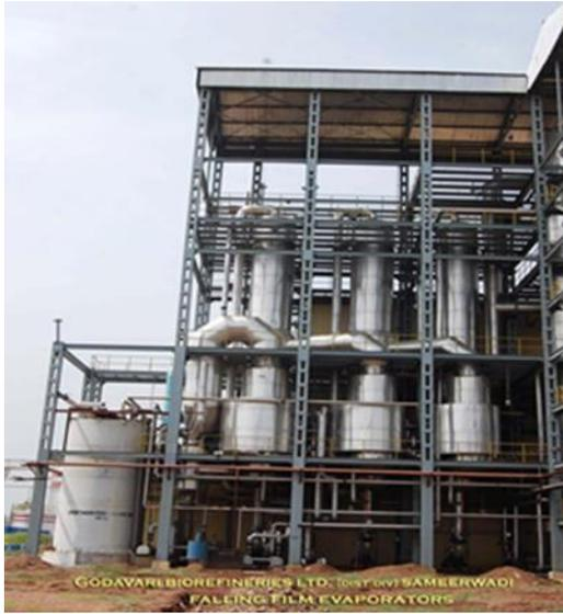
**I<sup>st</sup> Stage Evaporation (Falling Film)**
