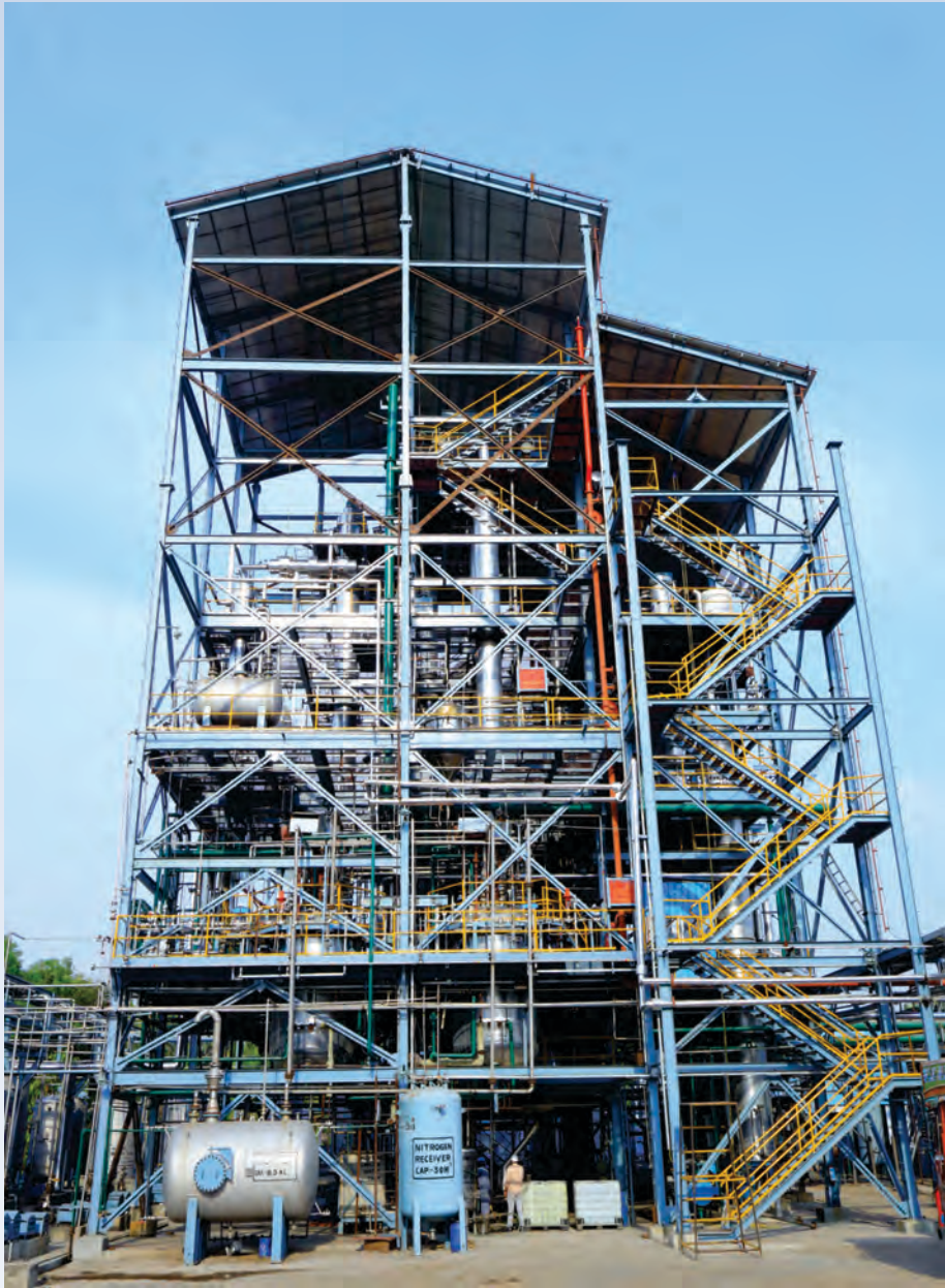
New Specialty Chemical Plant, Sakarwadi
