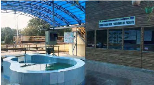
Figure 45: Effluent Treatment Plant
